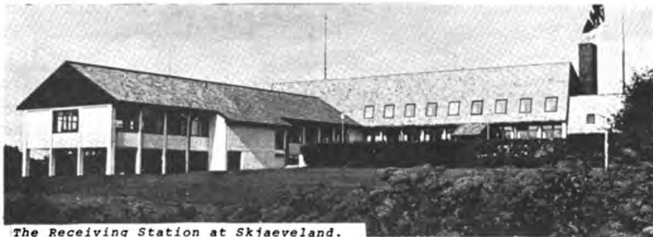
The Receiving Station at Skjaeveland.
